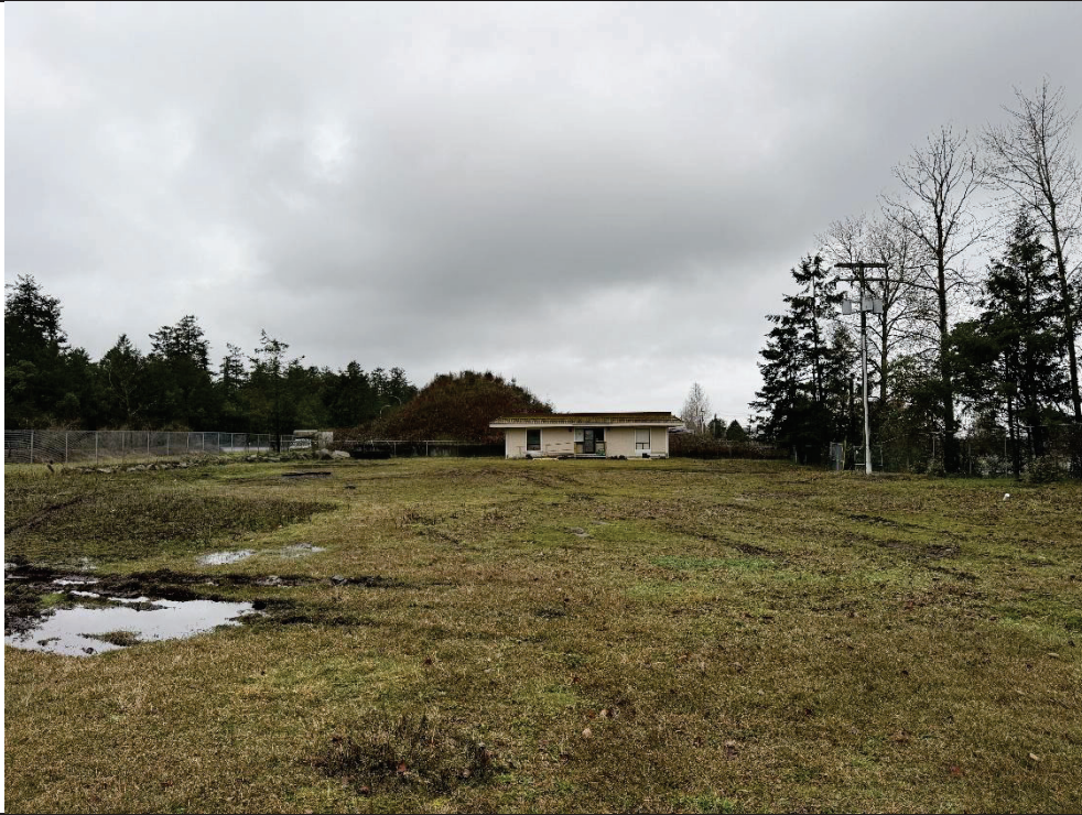
Office building on the North end of the property.
