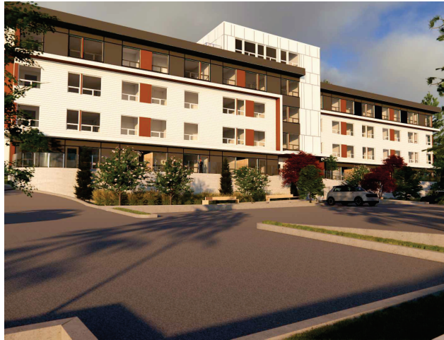
View from Back Parking Lot looking West
