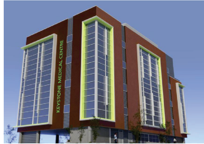
2 VIEW FROM NORTH-WEST OF BUILDING FRONTING DUFFERIN CRESCENT
