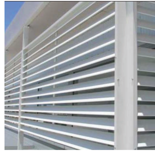
ROOF HVAC SCREEN
