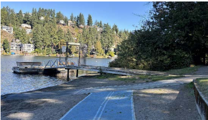
Figure 4: Accessible Fishing Dock Access and Mobi-Mat
