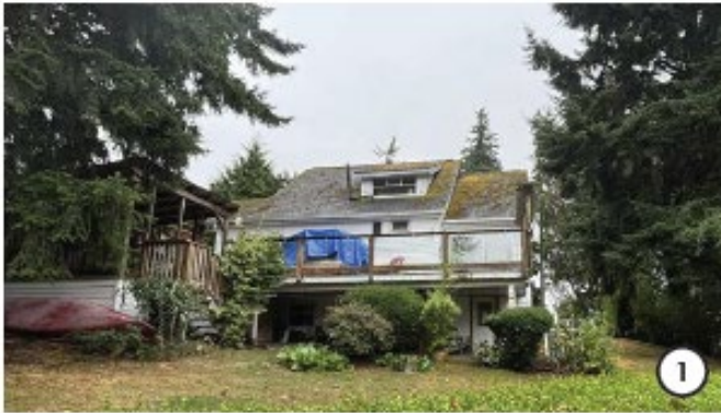
Figure 8: Acquired Property: 4288 Victoria Avenue
