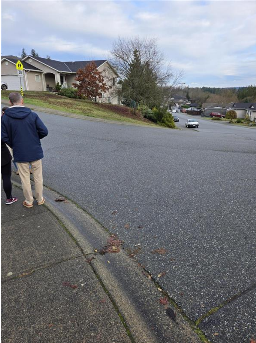
Figure 32 - Existing Width of Intersection at Montana Road/Ranchview Drive/Kentucky Place (Approximately 17 m)
