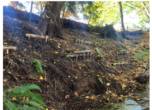
Bank stabilization along the Walley Creek corridor in Morningside Park.
