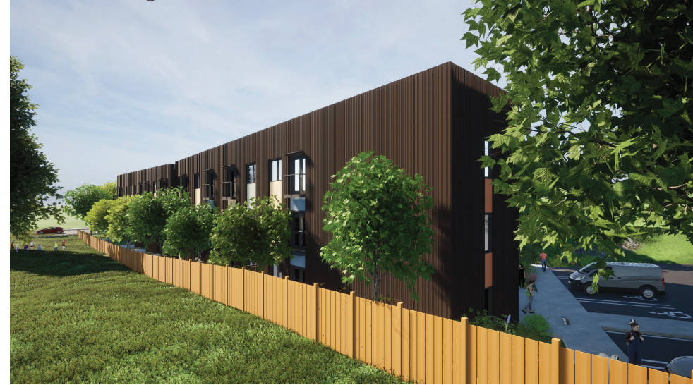
Building C from neighbouring yards to the north
