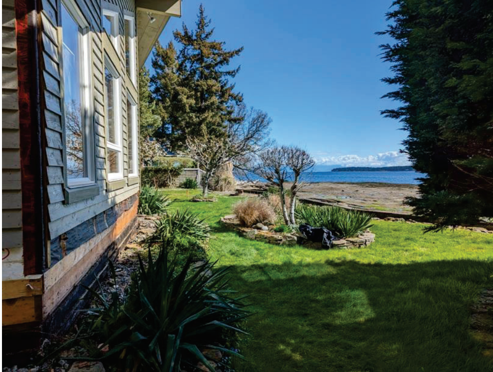
Photograph 1. April 9, 2024. View south – north along the east (oceanfront) side of the house.
