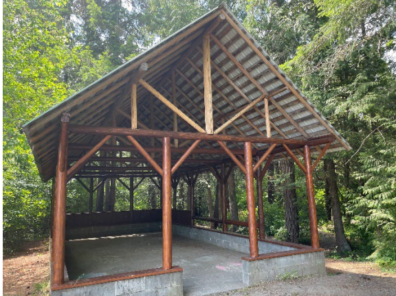
Photos of new reinforcements of the Errington Community Park pavilion and market stalls
