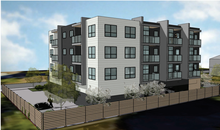
REAR VIEW OF BUILDING, EAST
