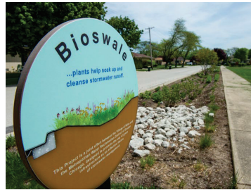
RAINWATER MANAGEMENT SYSTEMS / SIGNAGE ABOUT SUSTAINABILITY
