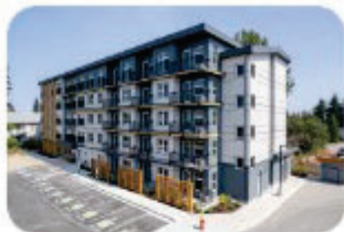
Sunfield Manor (1135 Seafield Crescent) 62 Homes - Affordable Housing for seniors and people with disabilities
