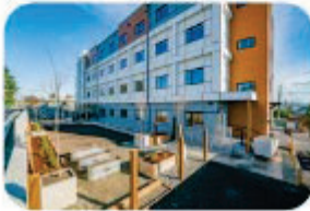
Samaritan Place, Supportive Housing at 702 Nicol Street, Nanaimo
