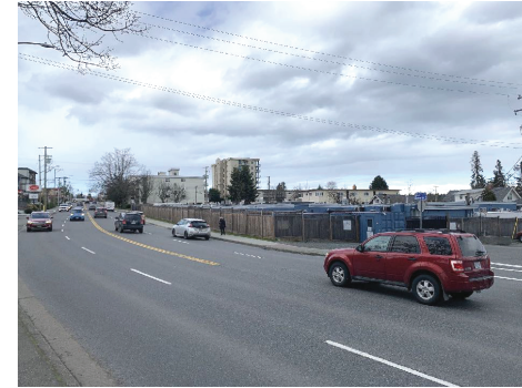
STREET VIEW FROM TERMINAL LOOKING NORTH
