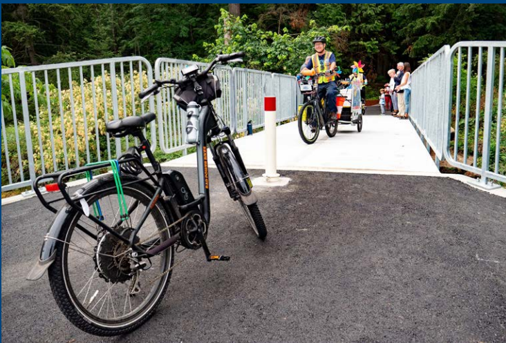
Lenhart Bridge Replacement
