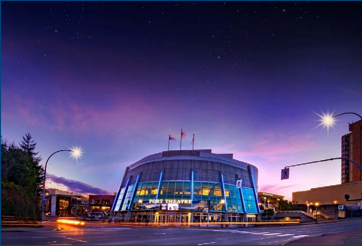
The Port Theatre - new roof
