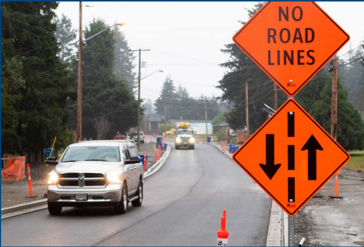
Metral Drive Complete Street Project
