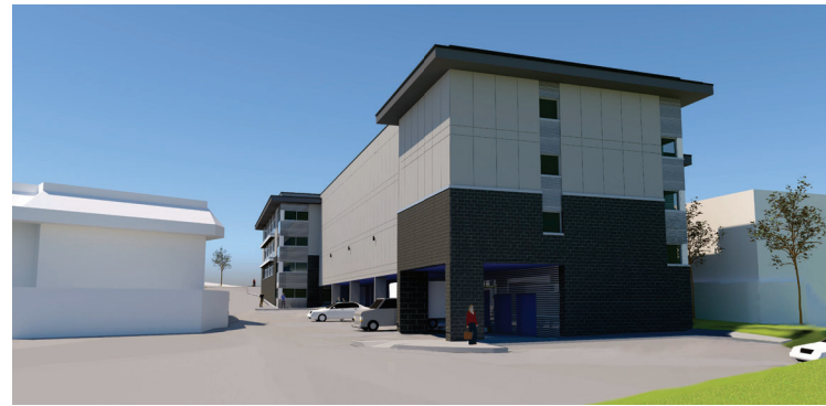
4 VIEW FROM NORTH-EAST
