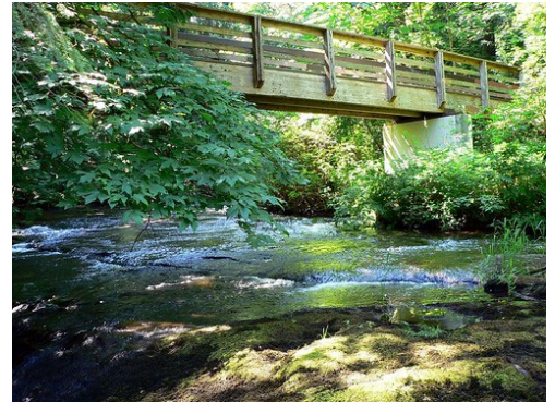
The Millstone River flowing through Bowen Park.
