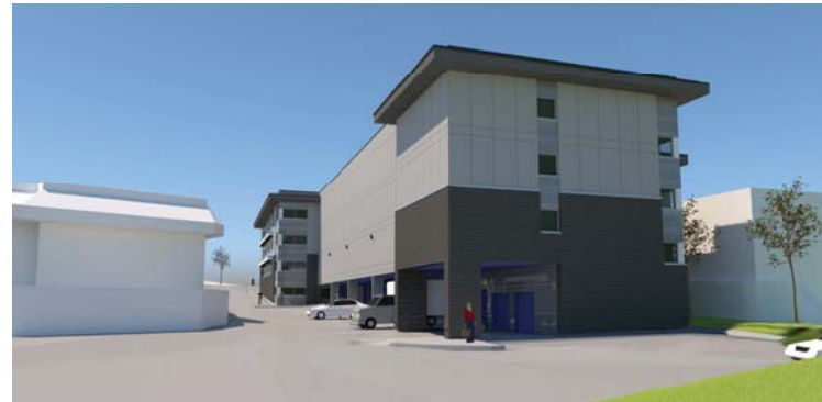
4 VIEW FROM NORTH-EAST
