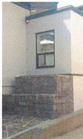
REVISION - DOOR & STAIRS REMOVED ADDED 3FT X 5FT WINDOW WITH 6FT X 4FT AND 1FT X 7FT TWO LEVEL STONE FACED PLANTER
