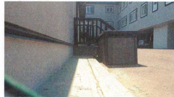
WESTERN ELEVATION PATIO ACCESS LANDING
