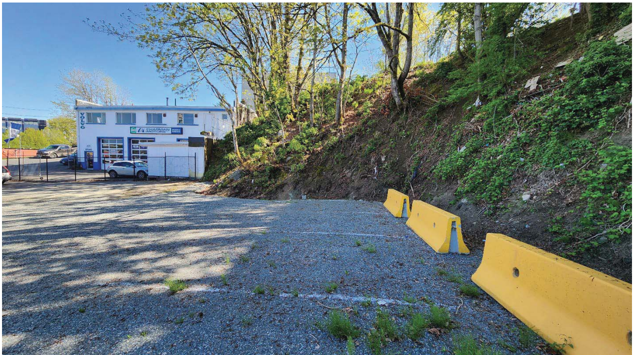
Adjacent property on Fraser Street (Volvo Auto Repair)
