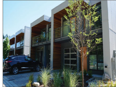
Image [above]: Completed rowhouse development in Nanaimo.
