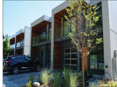
Image [above]: Completed rowhouse development in Nanaimo.
