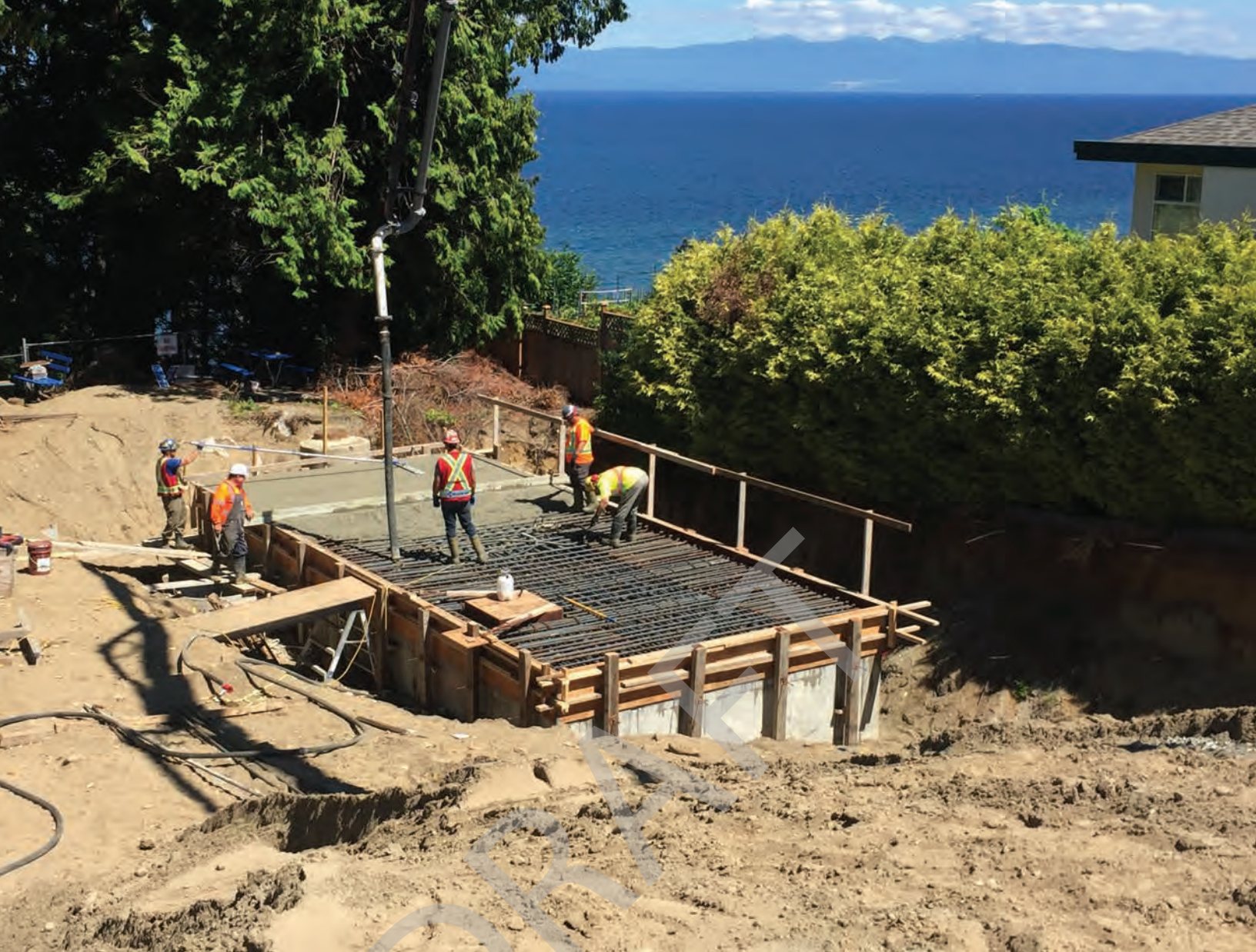
Concrete chamber built for Seabold Drainage project
