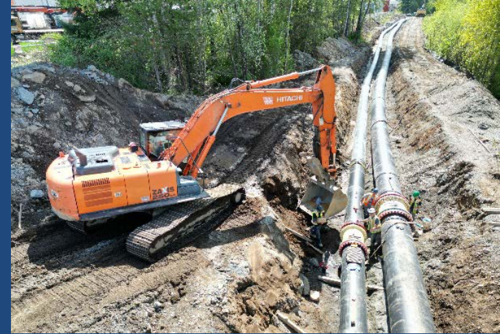
Midtown Water Supply Project
