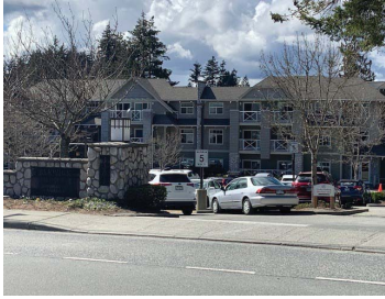
CURRENT VIEW AT DRIVEWAY ENTRY FROM ROSS ROAD
