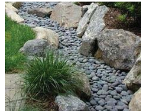
river rock channels/dry creek/ rain garden
