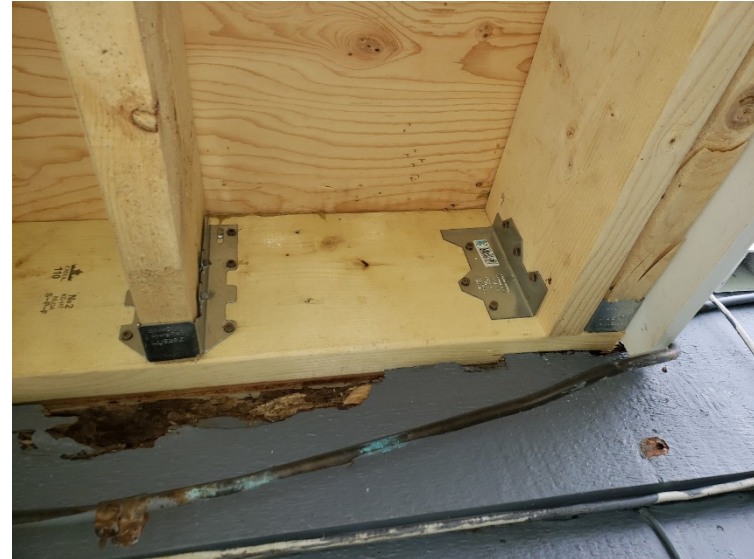
Joists are improperly installed with screws instead of nails. Screws have very little shear value.
