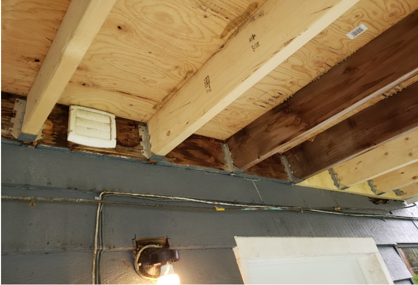
Joists are improperly installed with screws instead of nails. Screws have very little shear value.
