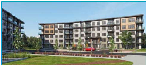
6985 Island Highway N.
