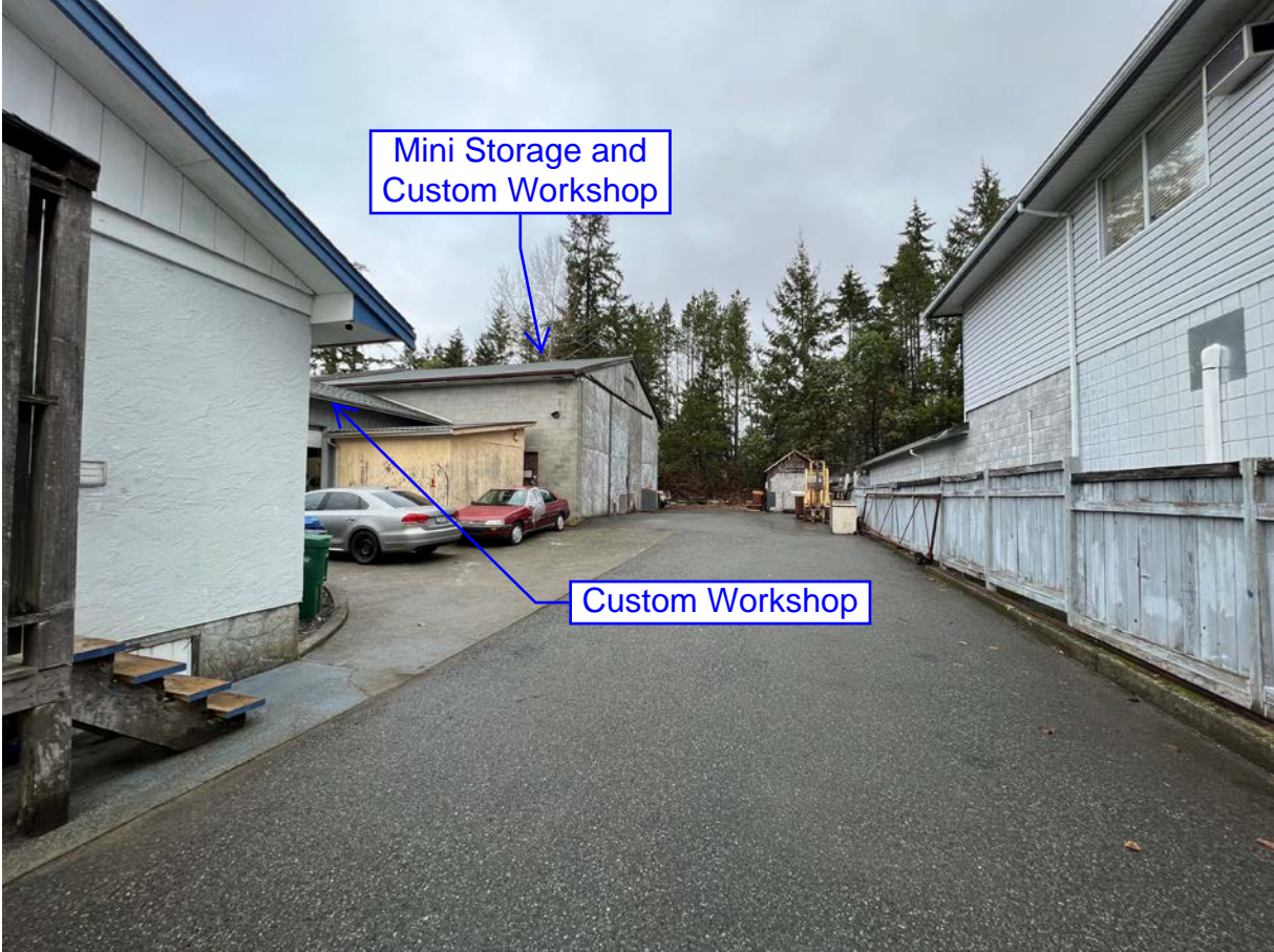
Existing Buildings on Subject Property (looking North from Driveway Beside Dwelling):
