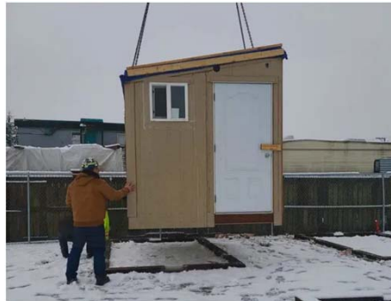
The Walyaqil Tiny Shelter Village in Port Alberni
