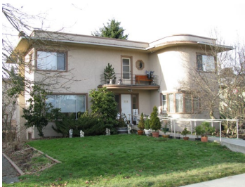
Name: York Residence Location: 908-912 Hecate Street Date: 1948
