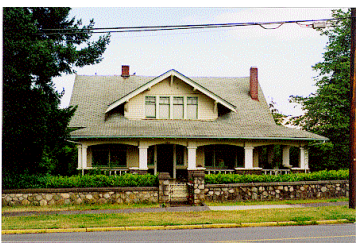
Name: Rowbottom Residence Location: 320 Machleary Street Date: 1913
