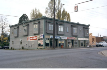
Name: Galloway Building Location: 405 Terminal Avenue N. Date: Circa 1920
