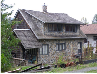
Name: Clements Residence Location: 420 Pine Street Date: 1929
