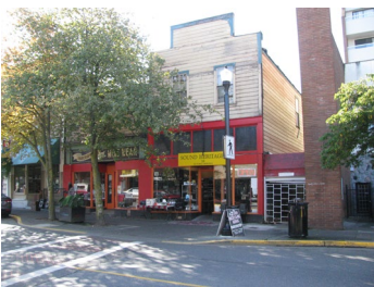
Name: Victoria Crescent Commercial Building Location: 33-35 Victoria Crescent Date: Circa 1892 or earlier
