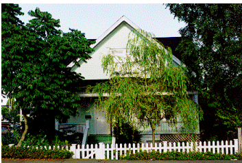
Name: Millstone Avenue Residence Location: 408 Millstone Avenue Date: Circa 1912
