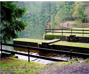
Name: Harewood Colliery Dam Location: 645 Wakesiah Avenue Date: 1910-1911
