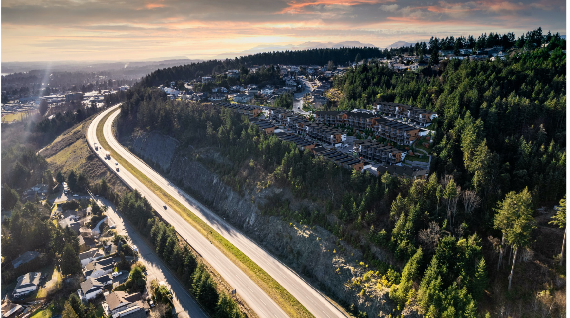
View Analysis - Nanaimo Parkway. Overview Looking West - Character & Tree Protection observed.
