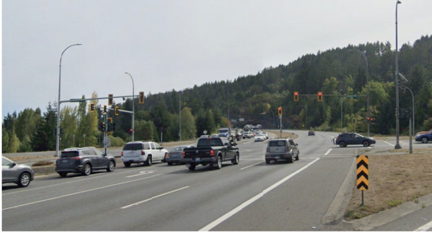
Pre Development: Jingle Pot Road + Parkway Looking South
