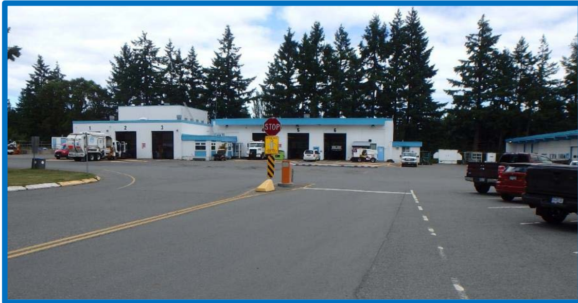
Image 10 Uncontrolled Main Gate Entrance
