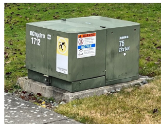
Pad Mount Transformer (PMT)
