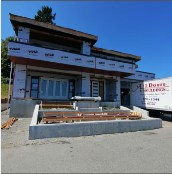
Photo 1: Looking west at the front of the new house from Battersea Road showing the subject retaining walls . The retaining walls allow for plantings to be installed within.
