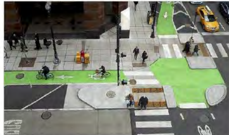
Intersection accommodating separated cycle tracks.
