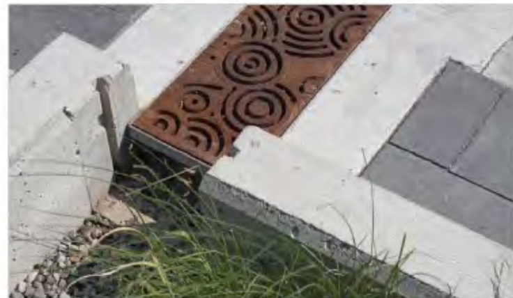
An example of public art integrated into the sidewalk and streetscape design.
