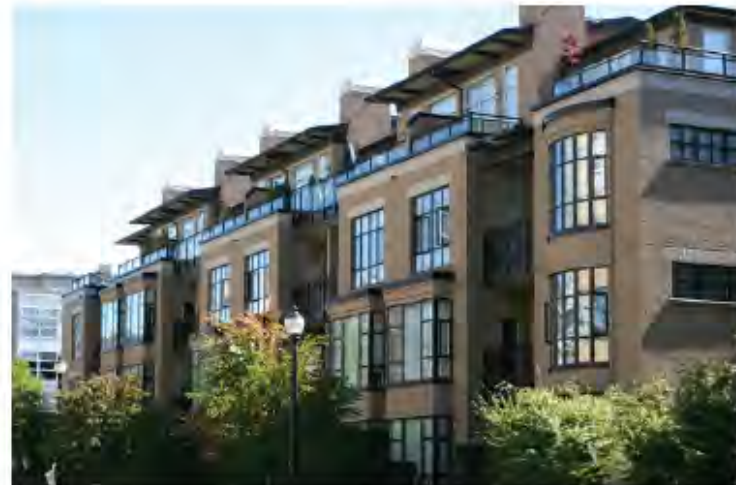
A building with a significant upper storey setback utilized as private balcony spaces
