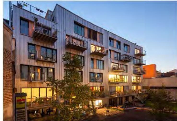
A high performance (Passive House, Step 5 equivalent) residential building with thermally broken windows and a low window-to-wall ratio
