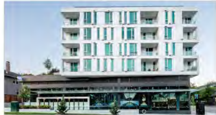
Building with higher at-grade transparency and lower WWR above
