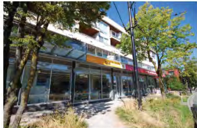
A high-rise building with a well-defined podium and an active retail frontage.
