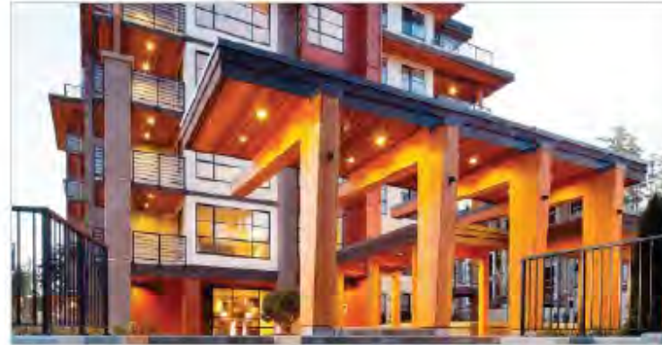
Utilizing and highlighting mass timber construction in a residential building
