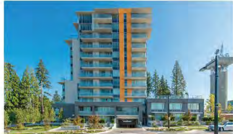
A high-rise building with a clearly-articulated podium, tower, and top.
