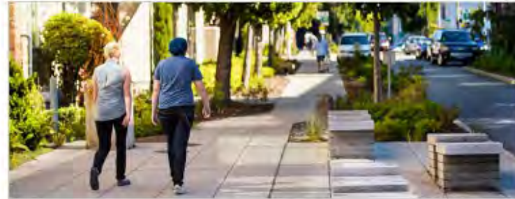
Sidewalk with integrated rain garden, street trees, and permeable paving
