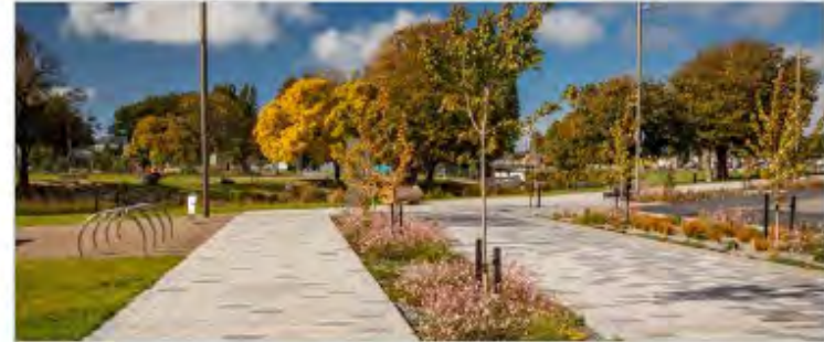
An example of permeable surfacing and soft landscaping area at the entry to a public park
