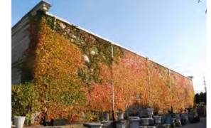
2. The creation of a green wall through the utilization of parthenocissus tricuspidata.
