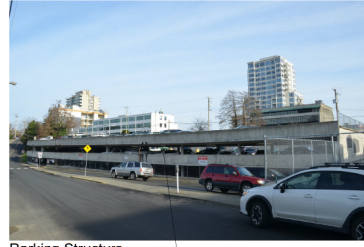
Parking Structure on Skinner St. (North Side of Site)
