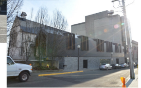
St. Paul's Anglican Church on Chapel Street (Across from Site to Southeast)
