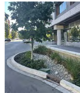
2. Street surface runoff collection into rain garden.
