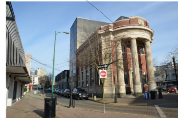
GNL Building at Church + Chapel Streets (Southeast of Site)
