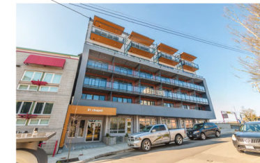
91 Chapel Street. Mixed Use. Studio NA on Chapel St. (South Side of Site)
