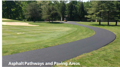
Asphalt Pathways and Paving Areas
