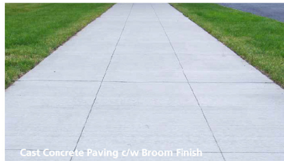
Cast Concrete Paving c/w Broom Finish
