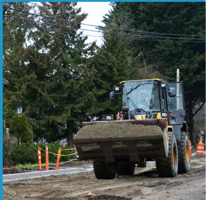
Metral Drive Complete Street construction
