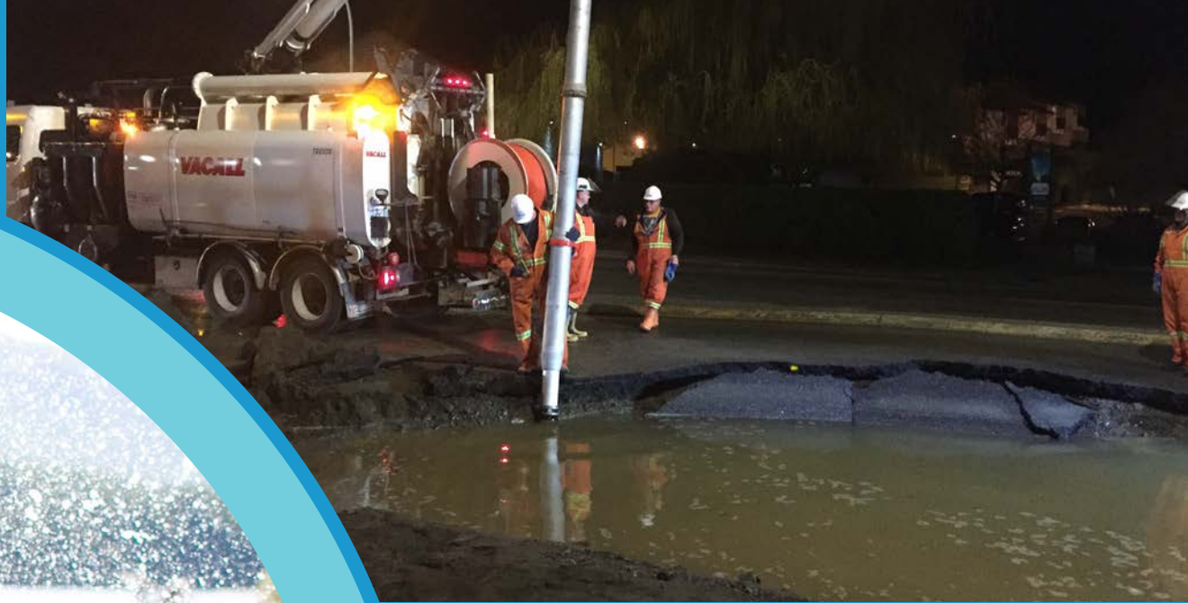
Crews repairing major watermain break on Bowen Road
