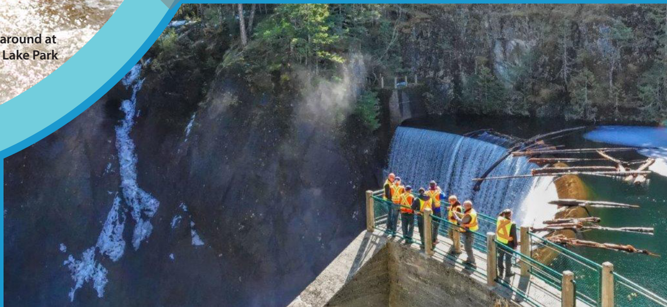
South Forks Dam
