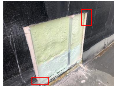
Photo 6: Location 3; new sheathing on the upstand wall was removed exposing a gap between the face of the spray foam and the backside of the sheathing (top right red rectangle, shown in Photo 8). Missing sheathing was also confirmed at the bottom of the recess (bottom left red rectangle, shown in Photo 7).
