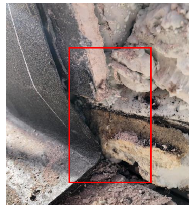
Photo 7: Missing sheathing at the base of the upstand wall. The new vapour retarder was not adhered creating a void the length of the upstand wall.
