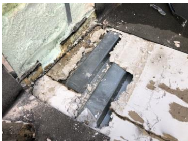
Photo 2: Location 3; deteriorated gypsum sheathing.
