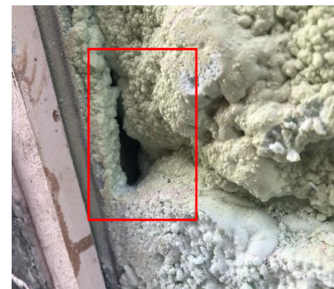
Photo 9: Void in the spray foam application. It is unknown how far the void extends.
