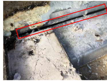
Photo 5: Location 4; sheathing shown in Photo 4 was removed on the right side of the photo exposing the gap outlined in red.
