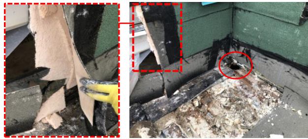
Photo 1: Location 1; Hole in the Q-deck circled in red, deteriorated gypsum sheathing on the surface of the roof and at the parapet. Inset shows damage to Phase 1 gypsum sheathing at the parapet wall.
