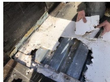
Photo 4: Location 4; deteriorated gypsum sheathing.
