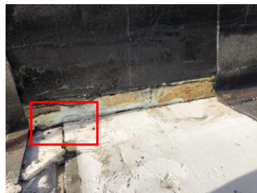
Photo 3: Location 4; deteriorated gypsum sheathing. Refer to Photo 5 for close up of indicated area.
