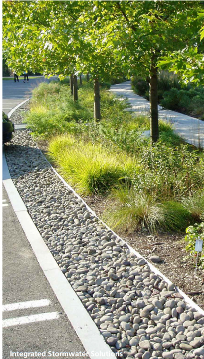
Integrated Stormwater Solutions
