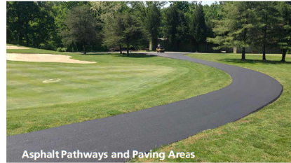
Asphalt Pathways and Paving Areas
