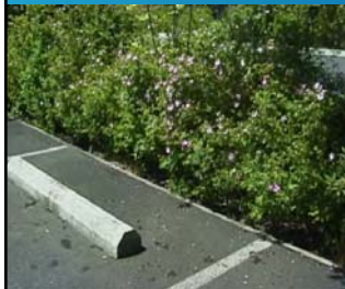
PARKING TO BIOSWALE
