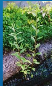
Live stake through soil wrap
