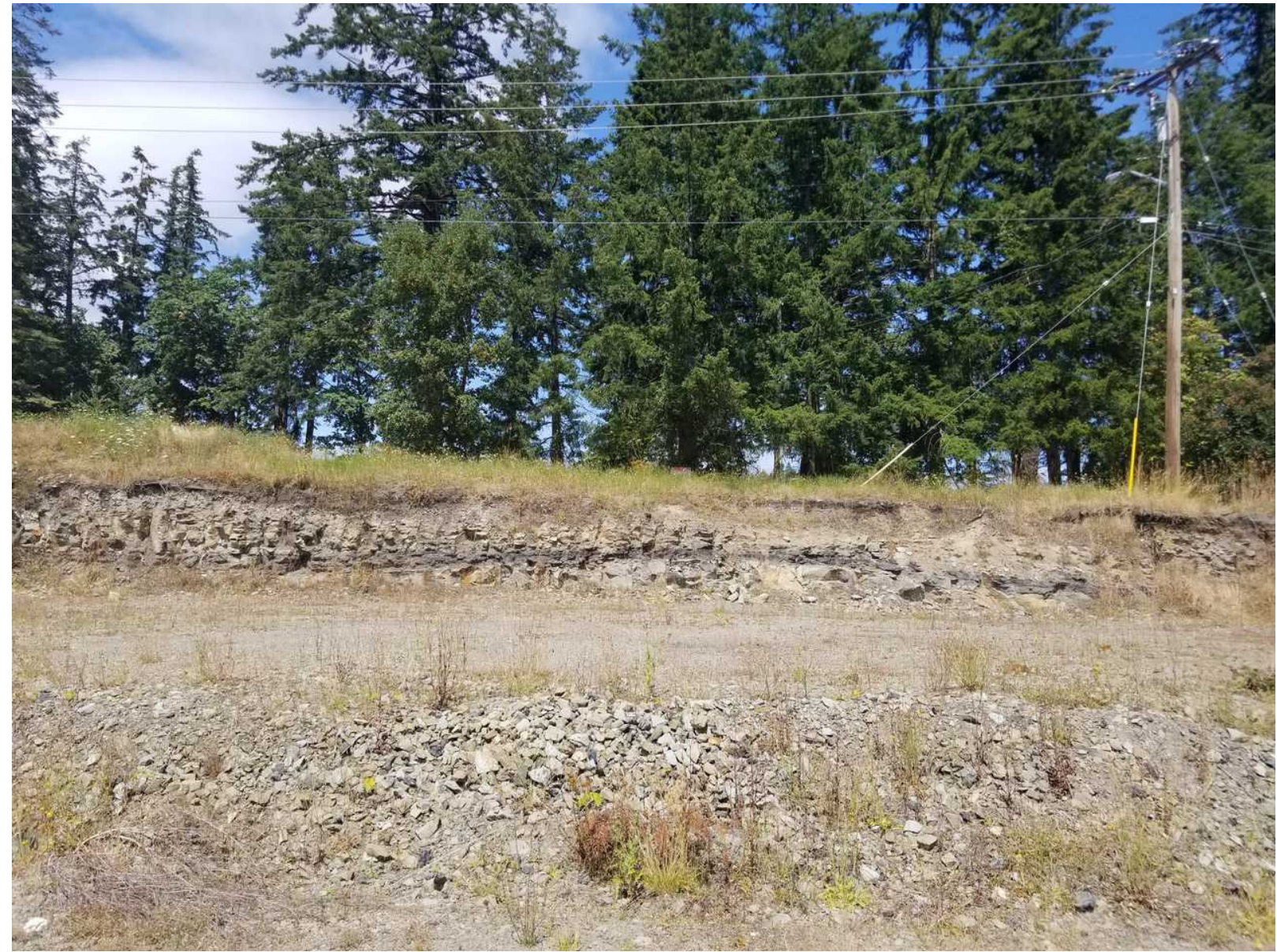
4063 Old Slope Road 2020-AUG-24 11:07
