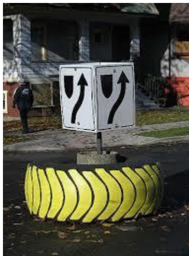
Figure 3 Example of Temporary Traffic Circle
