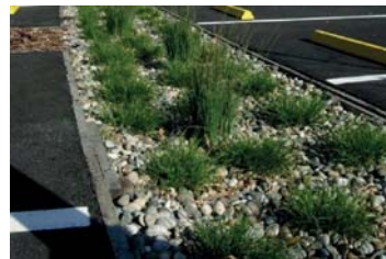
Armoured Swale Photo
