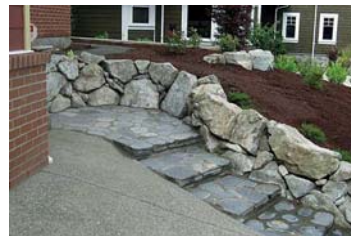
Boulder Retaining Wall Photo
