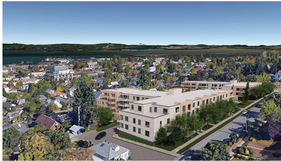
Machleary St. South West View
