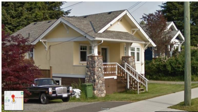
Photo 1 - view of South East corner of the residence
