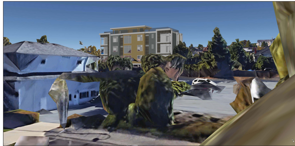
2 North-East Low View Note: - View from Wesley Street. - Image derived Google Earth 2018.
