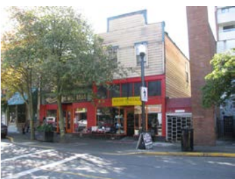
Name: Victoria Crescent Commercial Building Location: 33-35 Victoria Crescent Date: Circa 1892 or earlier
