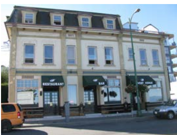
Name: Globe Hotel Location: 25 Front Street Date: 1887 (rear addition 1913) (side addition 1936)
