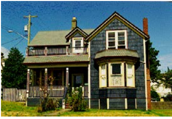
Name: McRae Residence Location: 98 Victoria Road Date: 1901
