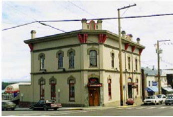
Name: Occidental Hotel Location: 432 Fitzwilliam Street Date: 1886-1887
