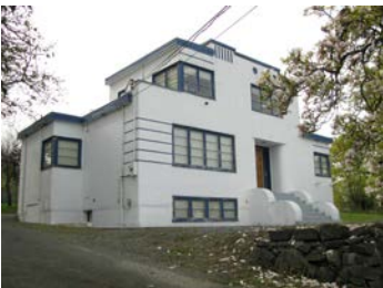
Name: Wardill Residence Location: 755 Terminal Avenue N. Date: Circa 1945
